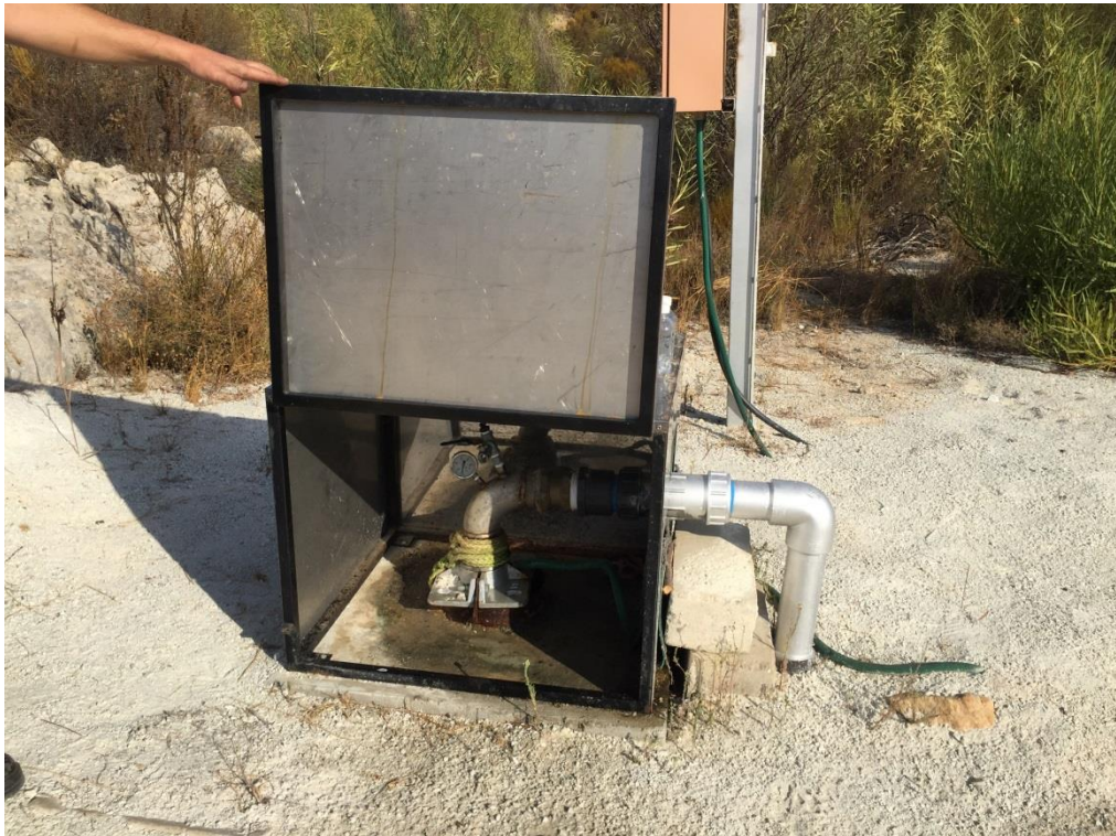
Photo 3: Stainless steel box, which is kept locked and secured on a concrete floor, preventing anything from falling or flowing into the production borehole. Note the sampling tap.
