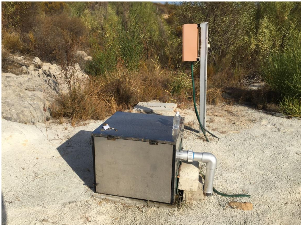
Photo 2: Secure stainless steel box surrounding the production borehole.
